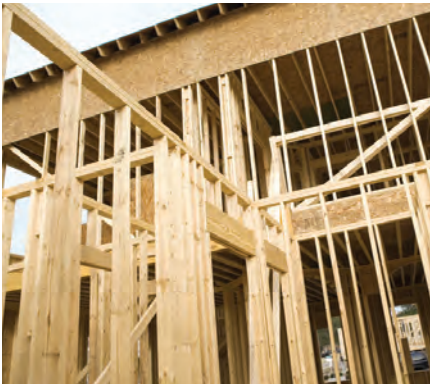
New Home Construction
